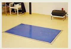
Lift table installed in a pit.
